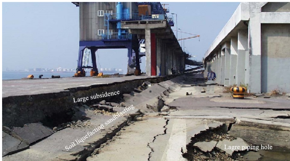
Figure 2. Damage to the rear line region of the pier caisson caused by the 1999 Jiji Earthquake, Taichung Port, Taiwan (Lai et al., 2007).
