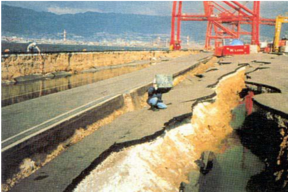
Figure 1. Damage to the rear line region of the pier caisson caused by the 1995 Great Hanshin Earthquake, Kobe Port, Japan (Kobe Geotechnical Collection, 2019).
